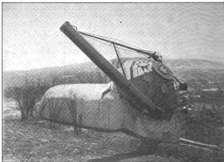
FIG. D WINTER VIEW TAKEN JUST AFTER COMPLETION OF GRADING, SHOWING NORTH END AND EAST SIDE
