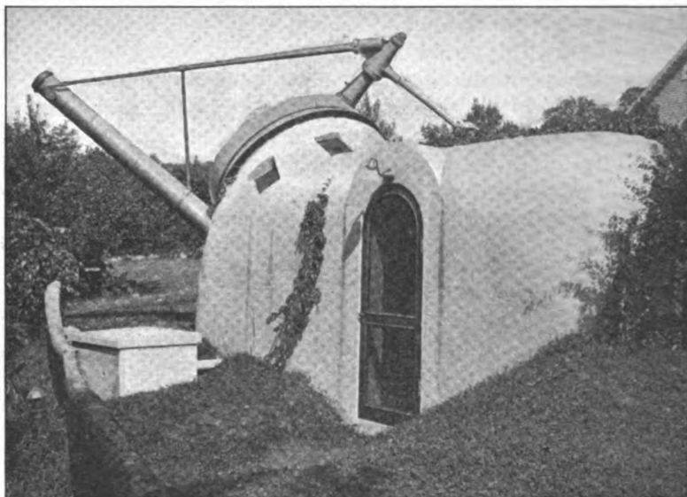
FIG. C VIEW SHOWING WEST SIDE AND SOUTH END
