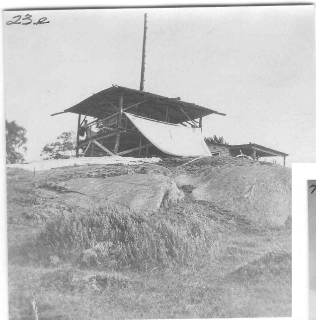
View to South
