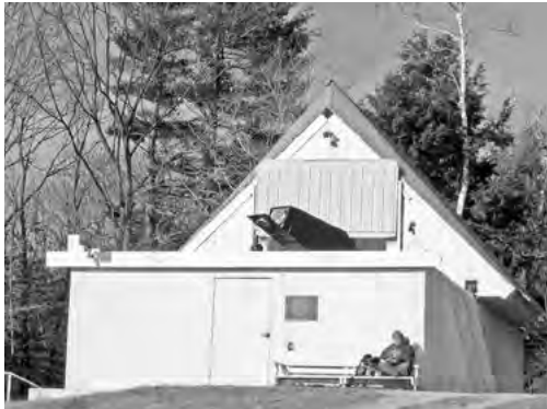
The McGregor Observatory with its roof retracted and the Schupmann telescope visible.
