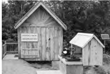
The beam from the objective lens enters the building via a tube through the wall, visible to the right of center on the building front.
