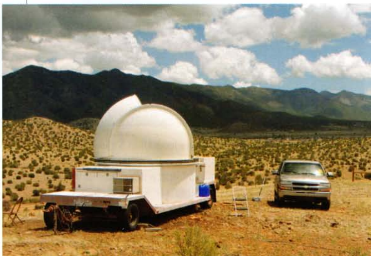
FOAH Observatory outside Magdalena, New Mexico, will eventually house several telescopes. The first installation is a 10-foot Parablum portable dome, surplus from White Sands Missile Range. A massive central section lowers hydraulically for three-point contact on the ground, leaving the telescope isolated from the large trailer. The current instrument is a differential image motion monitor for measuring astronomical seeing, a system originally developed for Apache Point Observatory and the Sloan Digital Sky Survey.
